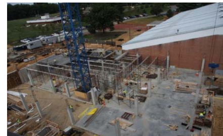
Figure 5: Concrete Placement, Sept. 15
